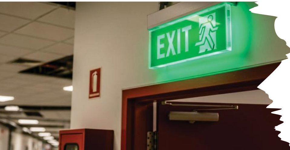
Emergency exits and firefighting equipment are basic safety requirements for all buildings
