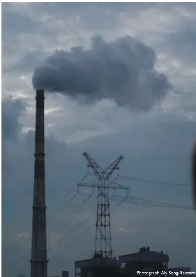
A coal-fired power plant in Shanghai. China approved more coal power in the first three months of 2023 than in the whole of 2021
