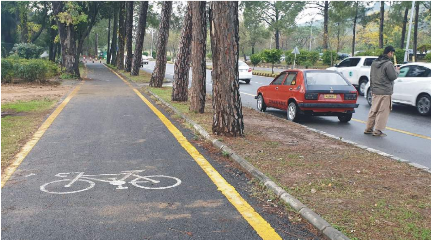
Islamabad Bicycle Lane Project is a network of 374 kilometers long dedicated tracks for paddle and e-bikes
